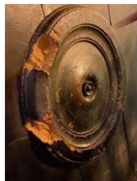
Fig. 7: Damaged Imperial Gate Photo: novasports.gr
